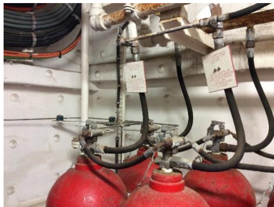
Image - Common arrangement of pilot bottles connected to system with flexible pipes
